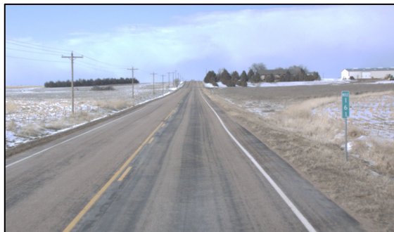
On the left is a stretch of Highway 76A near Keenesburg with Drivability Life of 17 years, or High Drivability Life. The photo on the right, in contrast, shows a stretch of Highway 59 between Sedgwick and Haxtun. The Highway 59 stretch represents a Low-Volume Highway with Drivability Life of nine years (Moderate Drivability Life). CDOT's system for managing pavement, which uses the Drivability Life metric, recommends a chip seal for this road in 2016.
