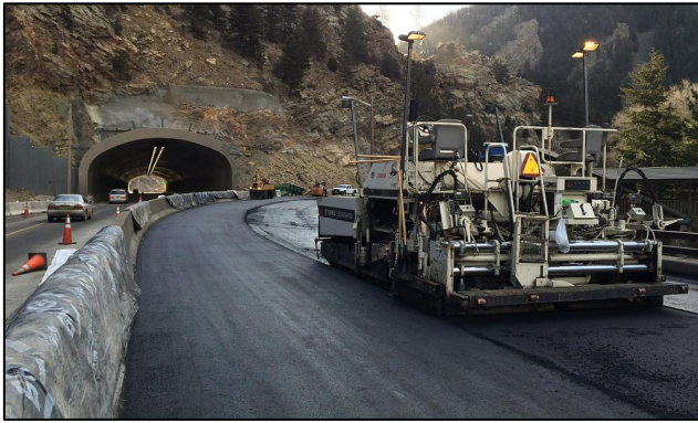
An asphalt paver places fresh, uncompacted asphalt pavement near the Twin Tunnels east of Idaho Springs.
